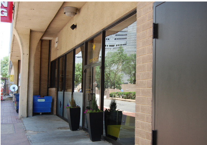
Entrance; looking east on Pacific Ave
