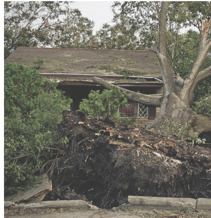
Hurricane Ike Storm Damage, Houston Texas
