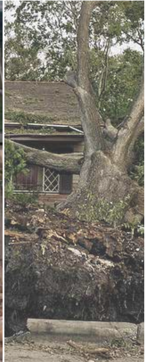
Hurricane Ike Storm Damage, Houston Texas
